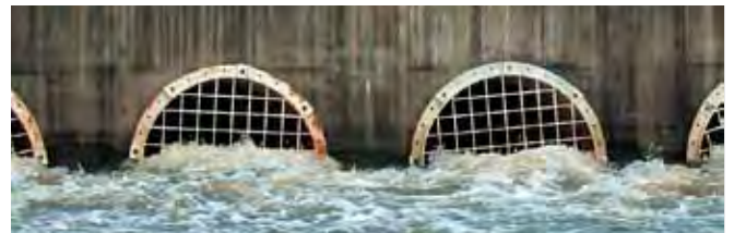
Balikera Pump Station, Grahamstown Dam.
