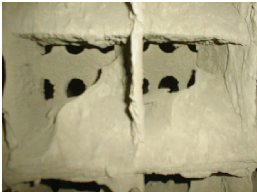
Ammonium bisulfate deposits at ESP inlet in a coal-fired boiler with ammonia injection for \text{NO}_x control.
