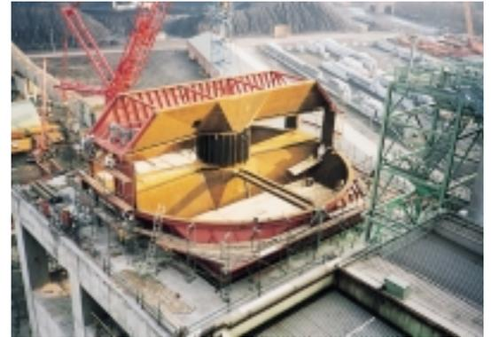
Erection of top cover with pre-assembled sealing plates
