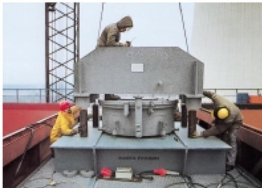
Support bearing and rotor lifting device
