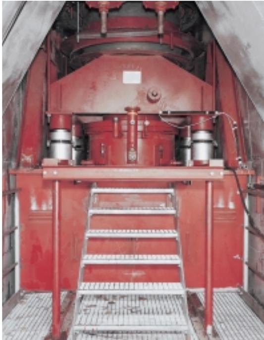
Rotor bearing and lifting device
